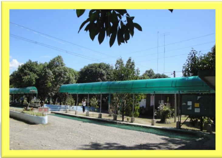
Newly constructed covered walk
