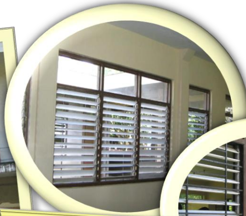
Repainting of Science buildings
