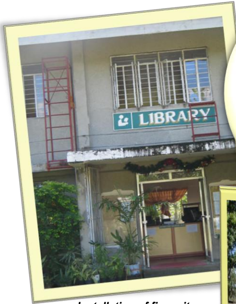
Installation of fire exits
