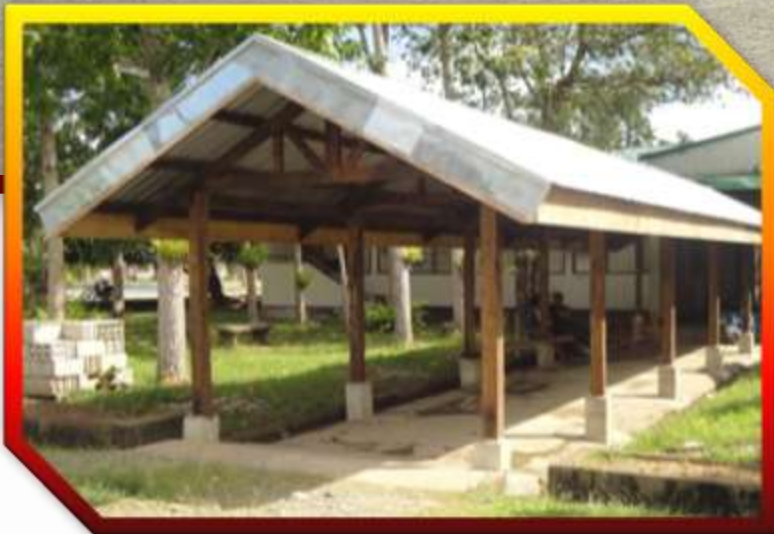
Covered Walk at CE Building
